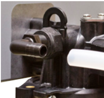
3.) Insert the backwash line onto the barb. It will be a snug fit. You will have to use a little force to get it all the way on.
