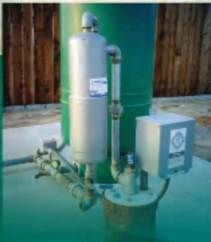
LAKOS Plum Creek Self-Cleaning Pump Intake Screens remove organic matter and debris from surface water, protecting an irrigation pump's intake.
