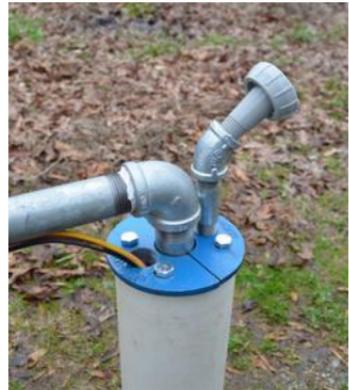
2 - Press the microphone tube into the small hole where the spout attaches. The tube should be long enough to reach through all of the fittings and reach approximately 1" into the well cavity. The tube can be extended up to 6ft. The tubing is 1/4" OD PE and is available at most hardware stores if additional tubing is required.
