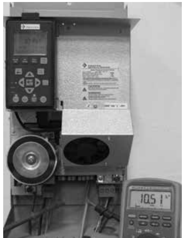
Figure 9. 40 PSI measurement
