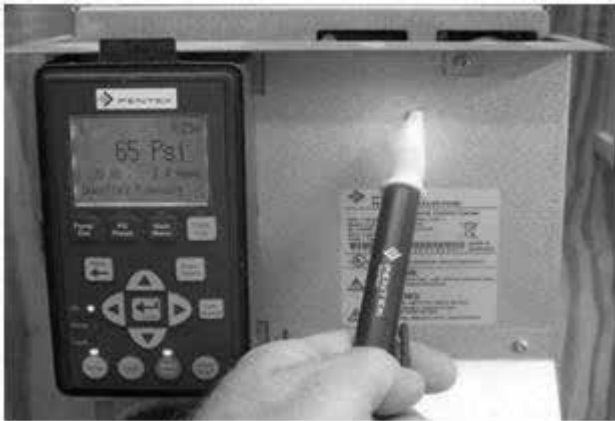
Figure 3. Easy ground check: Ungrounded
