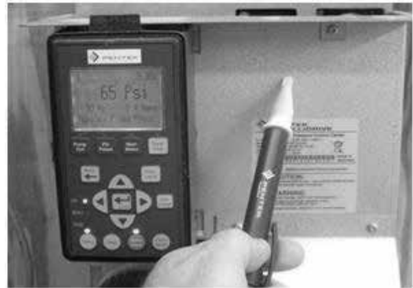
Figure 4. Easy ground check: Grounded
